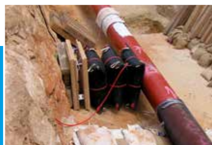
Lifting and leveling of pipelines - Construction -
