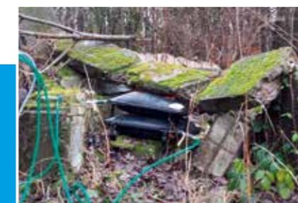
Lifting of blocks Stone, extrication - Civil Protection -
